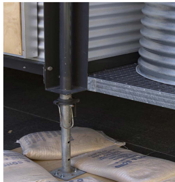
Figure 12: Variable height foundation [11].
