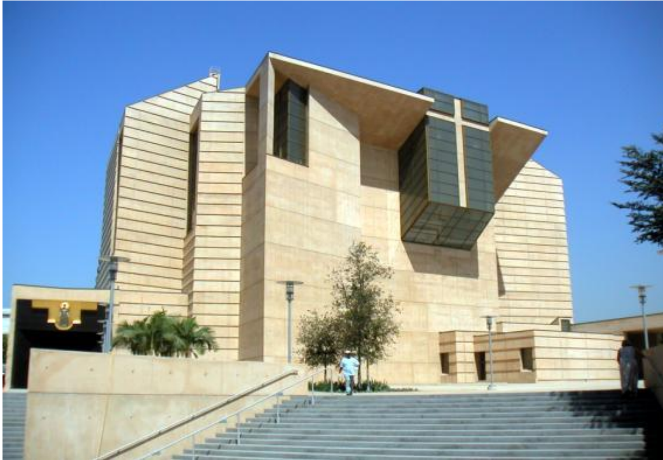
High density concrete with stainless steel reinforcement
