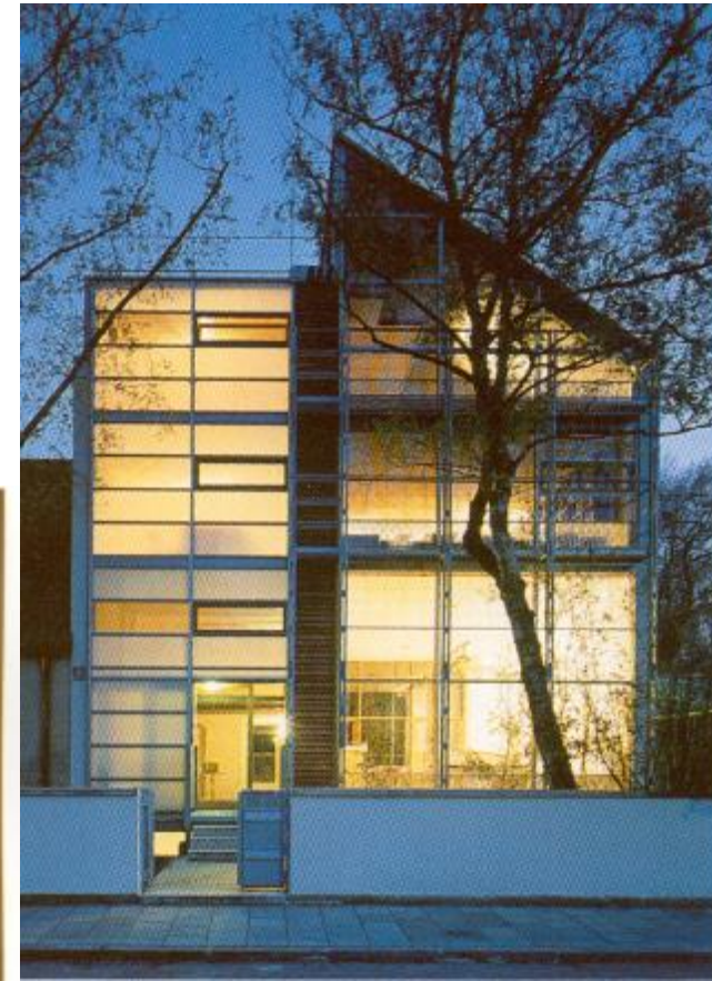
translucent walls with high thermal resistance
