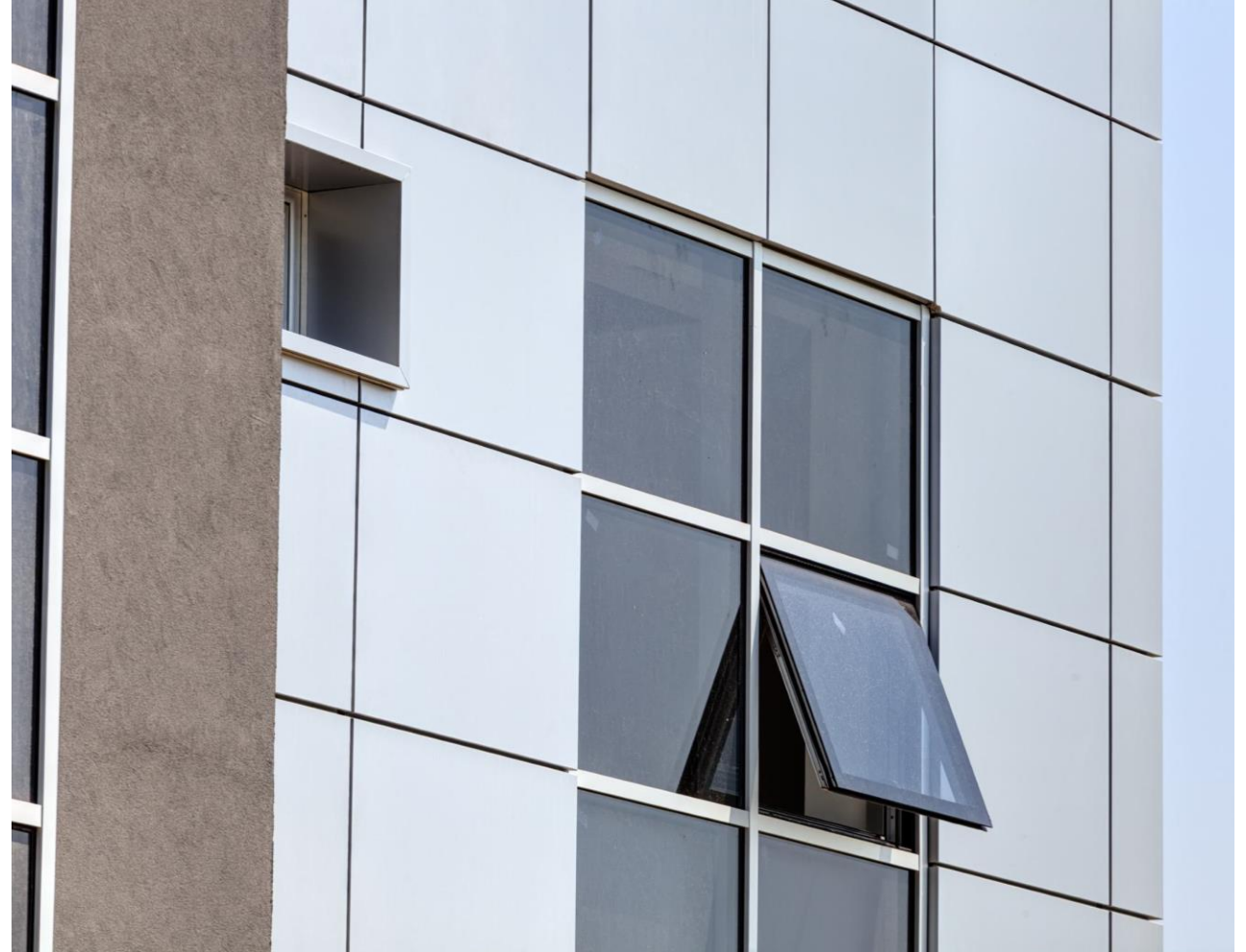
Aluminum composite panels used as building 'skins'
