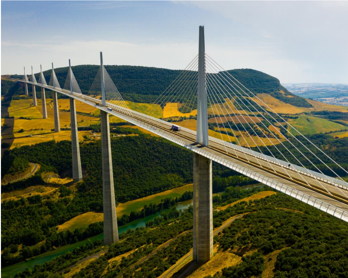
Millau Viaduct, France
