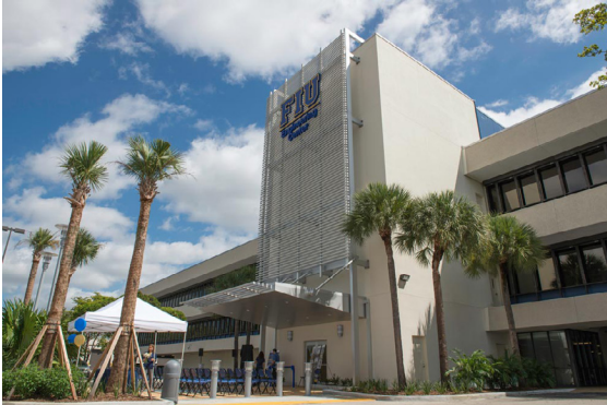
Figure 1: Florida International University's Engineering Center.
