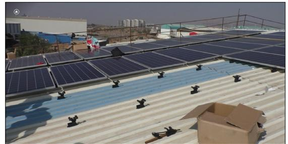
Indian commercial rooftop solar project installation using Tesserack™ Z. This picture shows that mounting hardware is installed in place for this solar panel row
