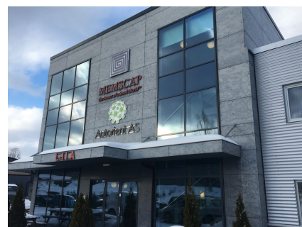
Autorient AS offices, Horten Municipality, Norway
