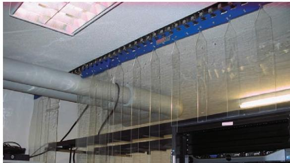
Once thermal partitions were installed in the data center, the room temperature could be turned up to save electricity and still maintain proper cooling for the equipment.
