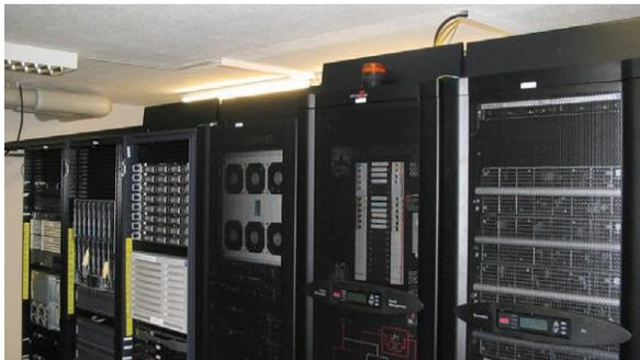
Server racks viewed from front of room. The three racks on the left house HPC servers. Ideally, cool air from wall-mounted air conditioners on the rear wall (behind the racks) gets drawn into the racks, and hot air from the servers is expelled out the front. Racks to the right of the HPC servers contain mid-range conventional servers, backup server, data storage units, file server and an uninterruptible power supply.
