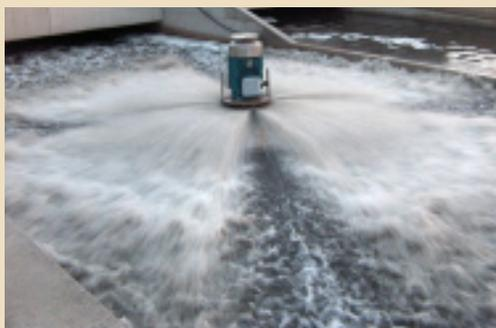
The surface aerator of this bio-reactor is used to resuspend the solids bed from within an aeration lane and to entrain air into the reactor.
