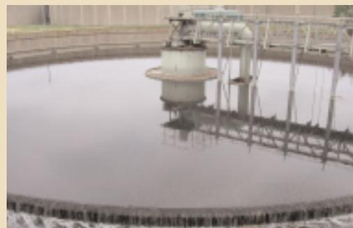
Activated sludge is settled out in this clarifier. Flow enters the tank from the top and flows radially outward.
