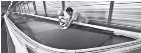
Starting the build: laying out honeycomb core material hull mold at Decision SA, Switzerland ©Carlo Borlenghi/Alinghi.
