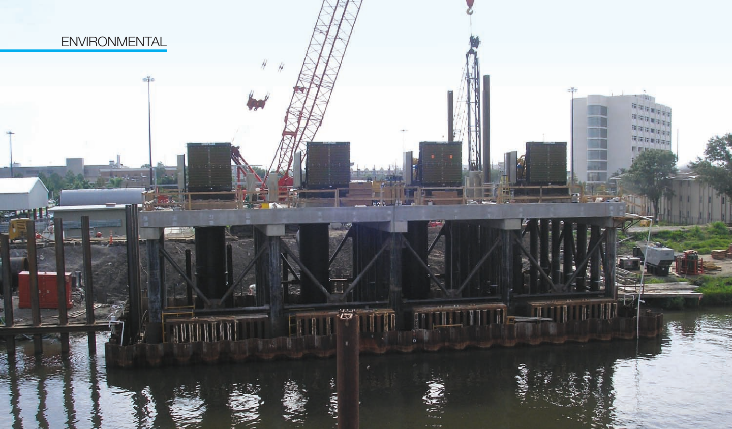
One of the four-bay New Orleans canal platforms under construction
