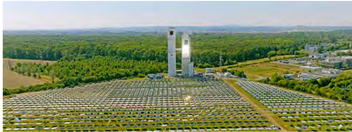
Aerial view of the solar tower and mirror field of DLR, Jülich. The mirror field concentrates the solar radiation onto the solar tower and heats up the solar receiver. Image courtesy of Synhelion.
